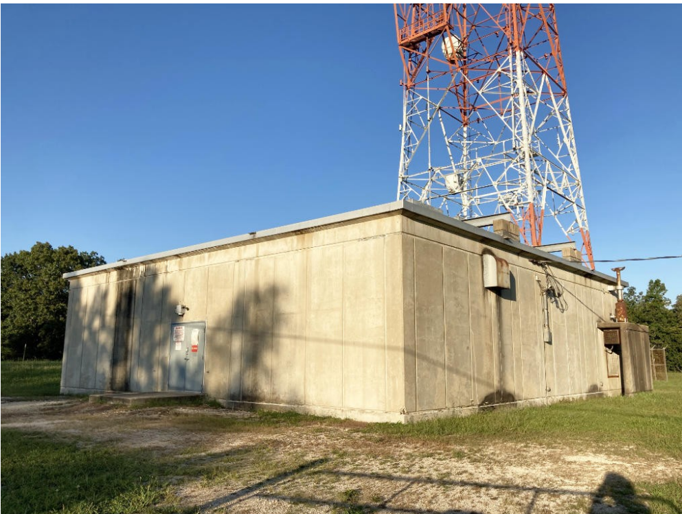
Semi-hardened (2 PSI overpressure) concrete base station with blast shield seen along right edge.
