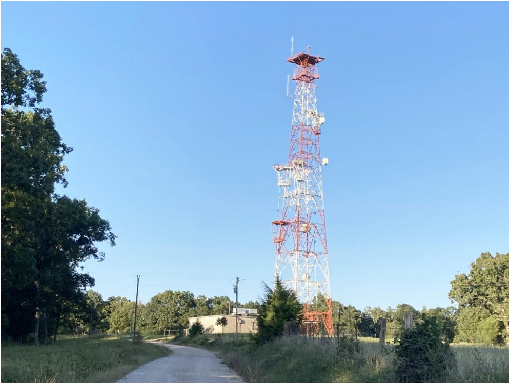
Site seen from the southwest on Maries County Road 613. The site's original horn-reflector antennas have been removed to make way for dipole array antennas (seen at and near the top of the tower) and shrouded parabolic reflectors used by the MOSWIN public safety radio system.
